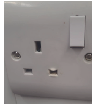
Fig 5. Damaged socket
